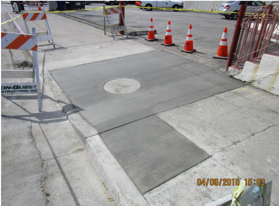
New manhole on Estudillo Ave adjacent to Galvan's Market
